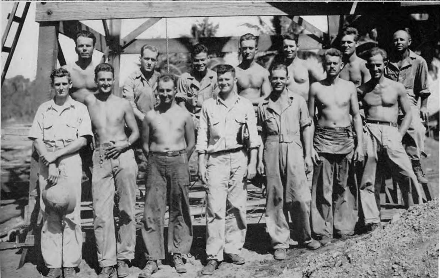
Tower Construction Gang
