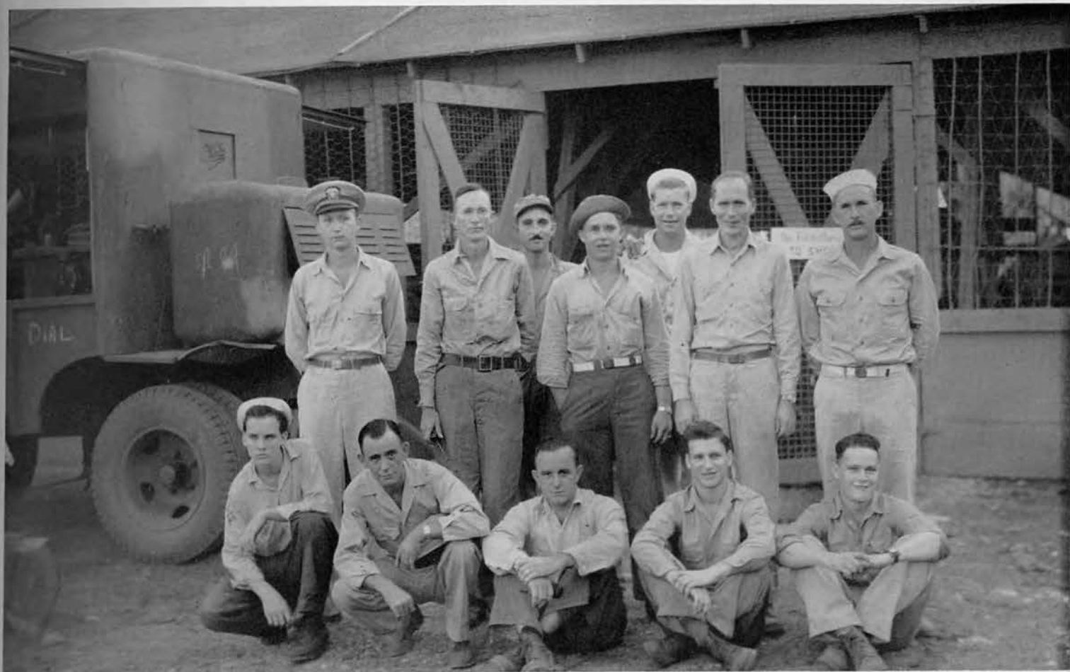
Electric Shop, Guadalcanal
