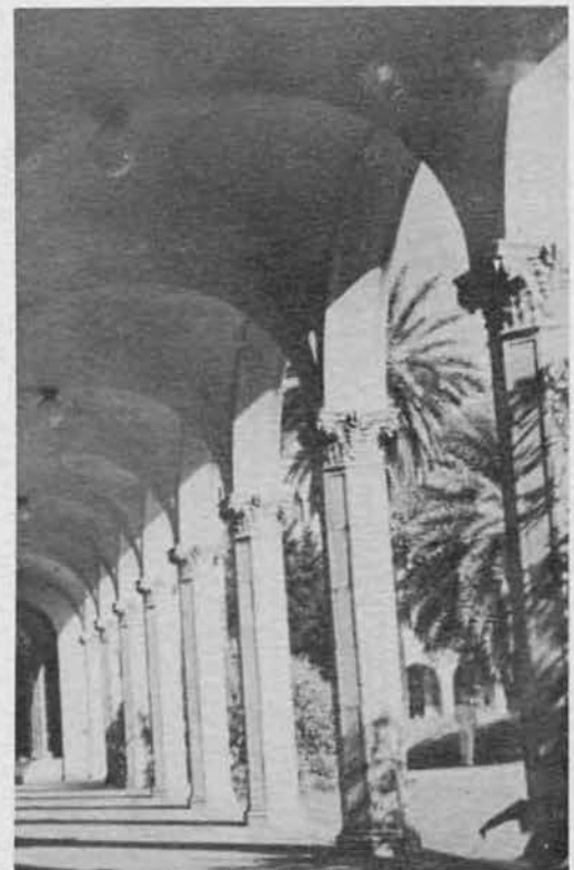
Outdoor Corridor, Federal Building
