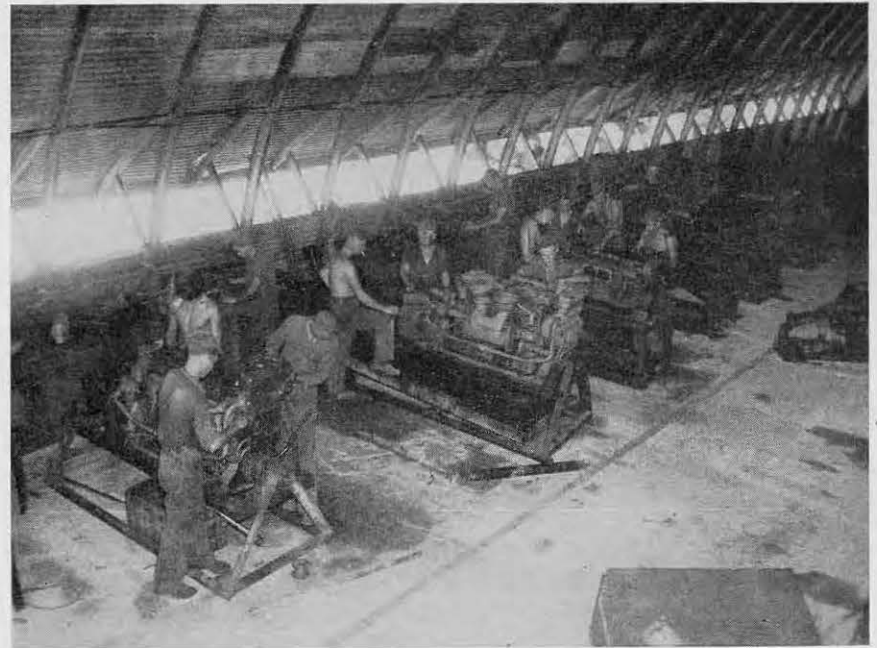
Diesel motors under repair in the new shop
