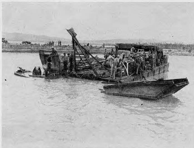
The barge is hoisted to the surface
