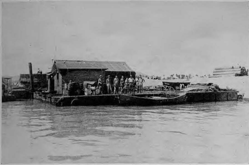
Here the engineers barge is tied up to a dredge made shore
