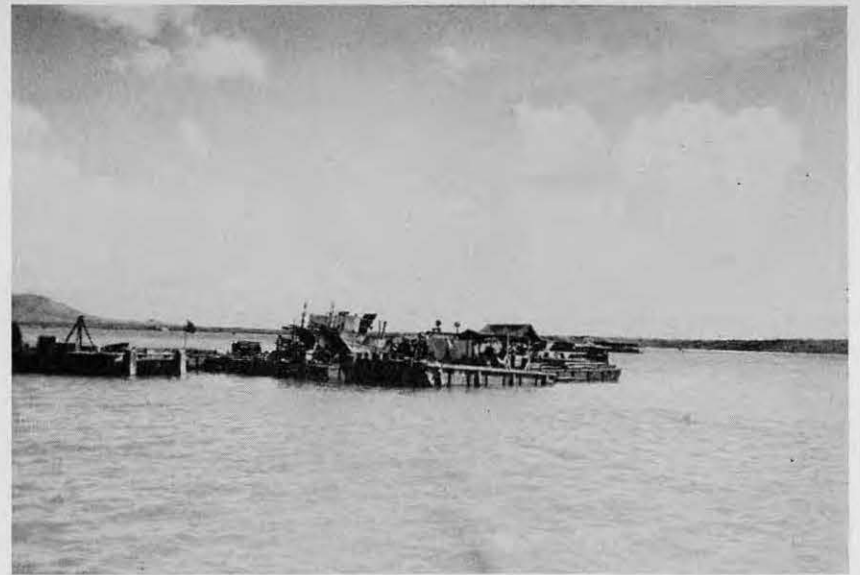
Another early view of the repair barges
