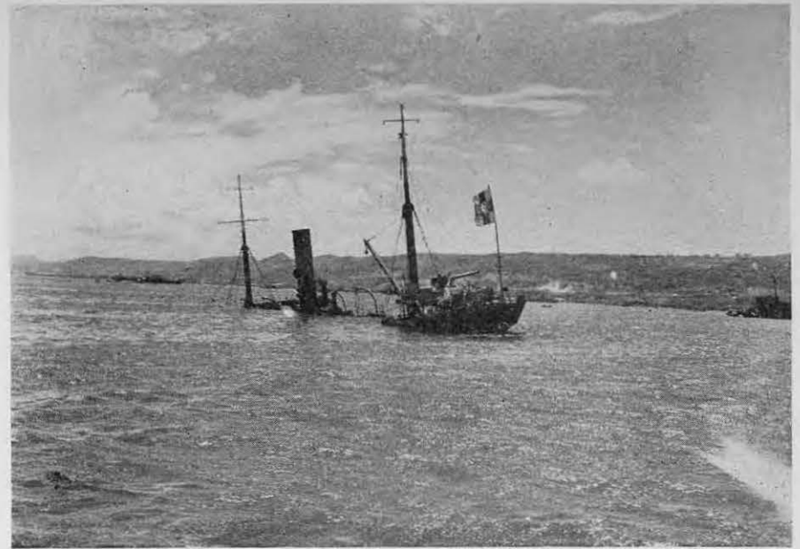
This hindrance to navigation was removed by blasting
