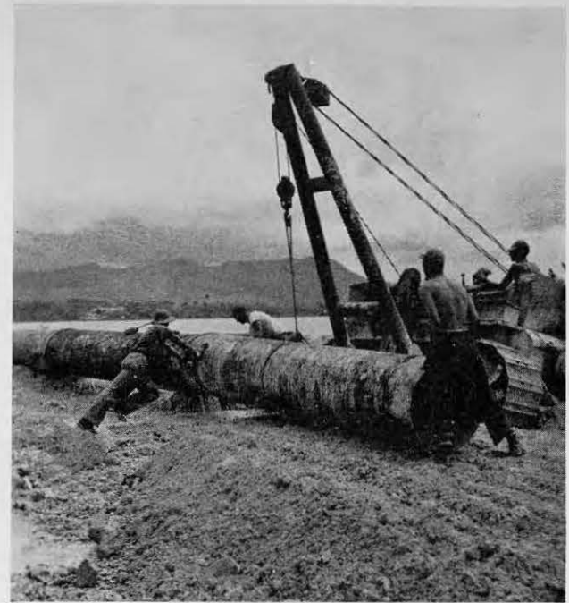
Assembling shore line for YM-21
