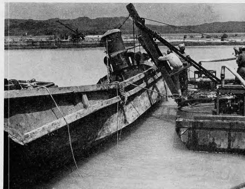
It is pumped out and the bottom patched
