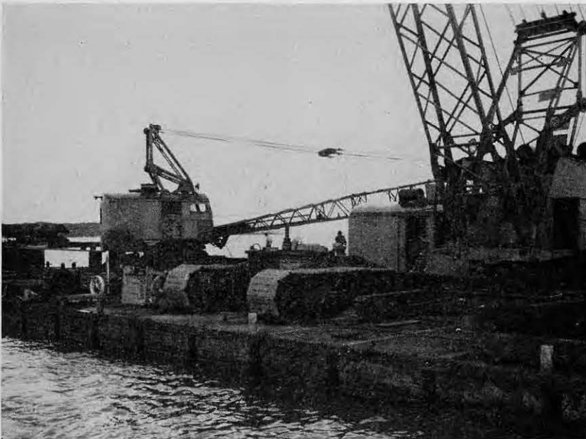
Whirleys undergoing repairs
