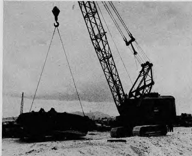
An 80-D lifts a huge pontoon, ready to float it
