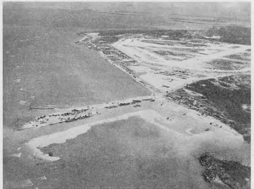
Nearly Completed Channel and Docksite
