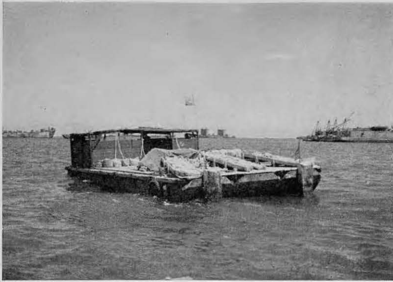
The planning and ingenuity of the powder crew resulted in this self-propelling preparation and placing barge
