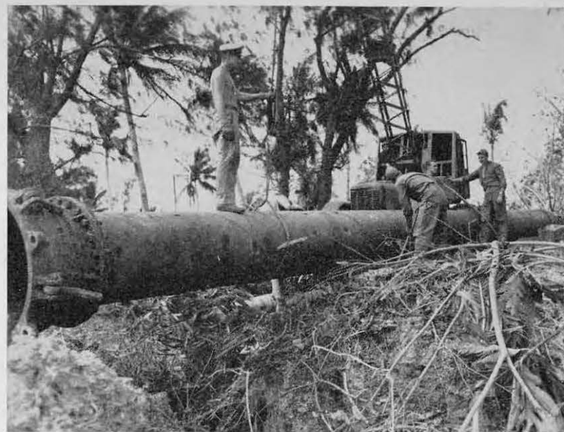
Placing a landing pipe
