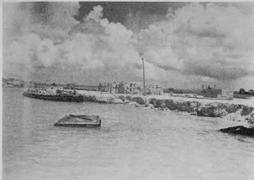
The piles of dynamite before the blast
