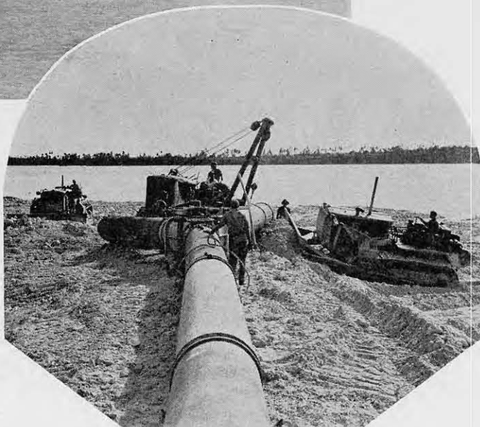
A "Y" is assembled on the fill
