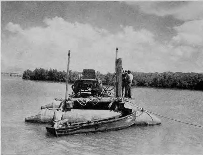
A fire engine on pontoons, for jetting borings made by the "Alligator"
