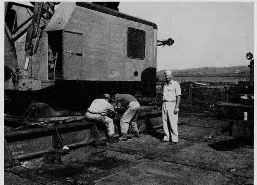
Carp Foltz supervises a repair job
