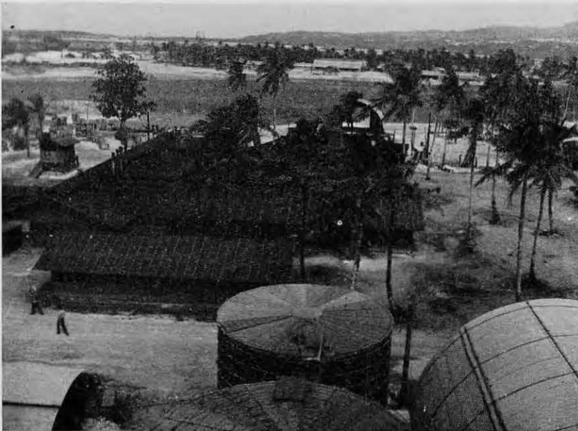
Exterior of the new mess hall
