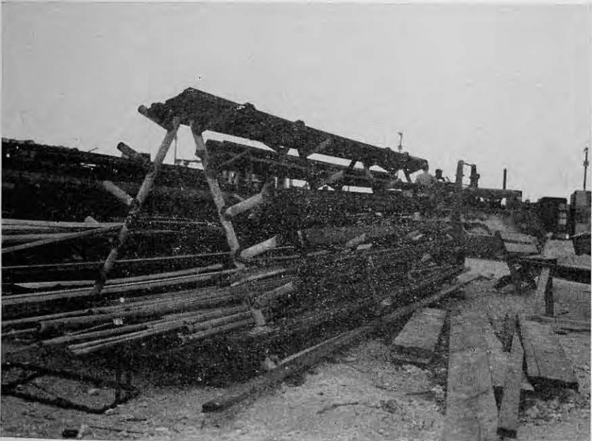
A home made pipe rack
