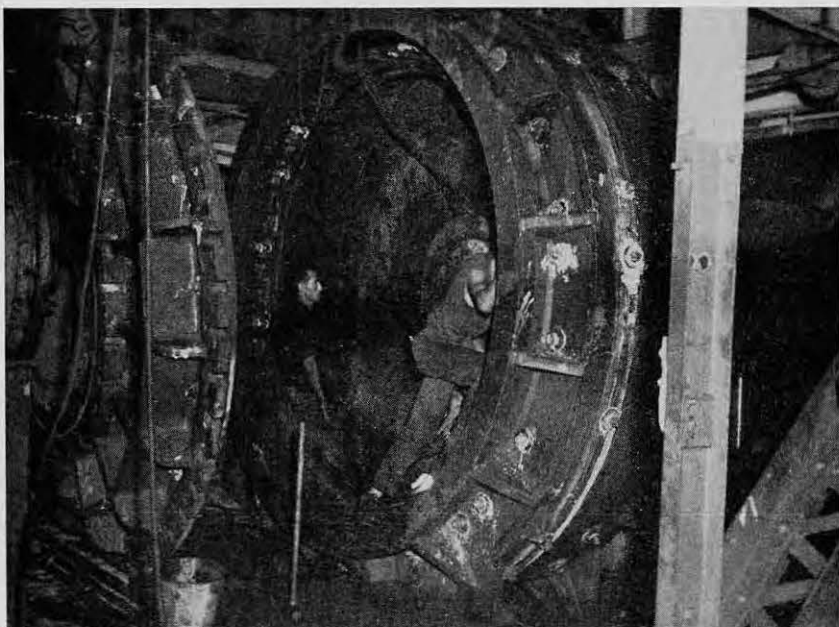
Take a look at the size of that pump, a mere bagatelle for these experts
