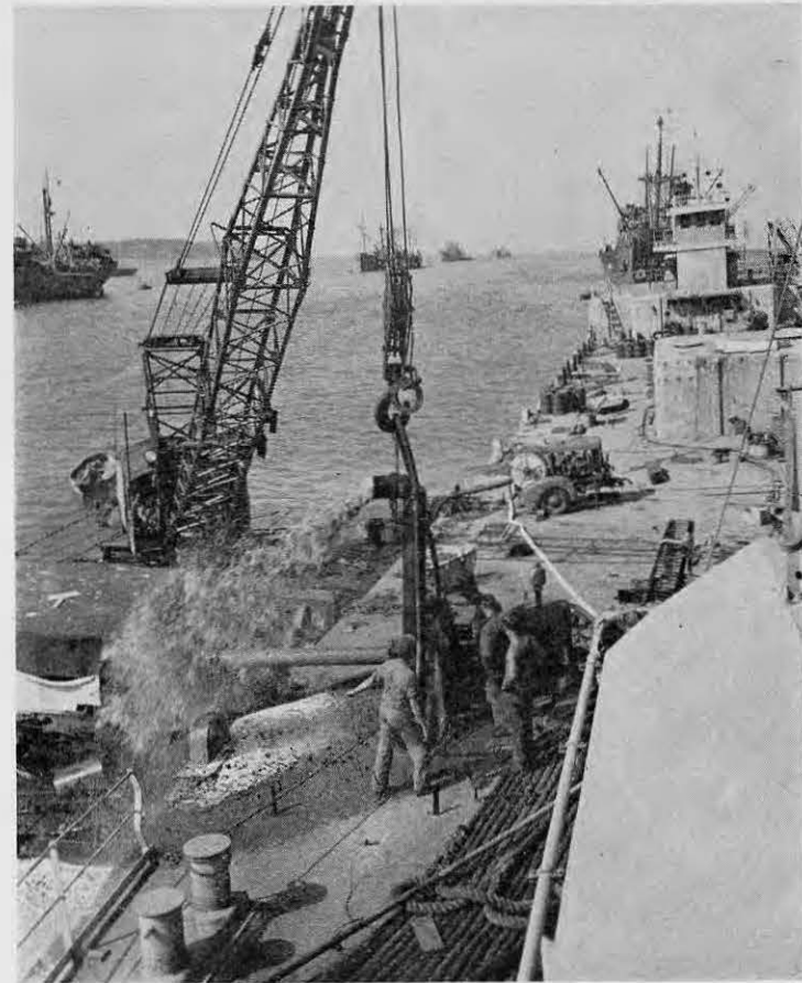
The gravel ballast is sucked out, with 301 Ingenuity
