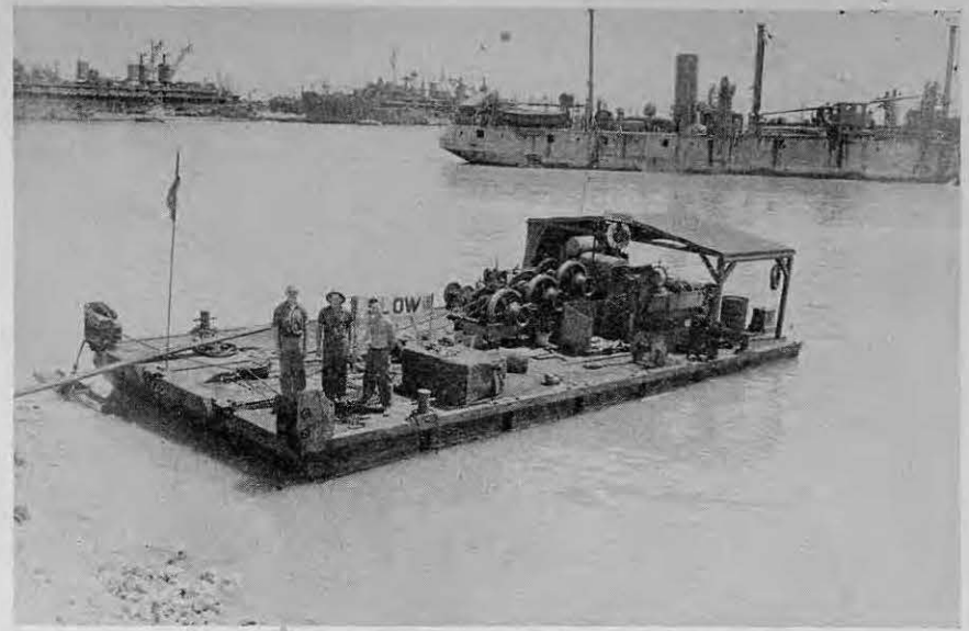
The beam drag barge, to knock the tops off those coral heads
