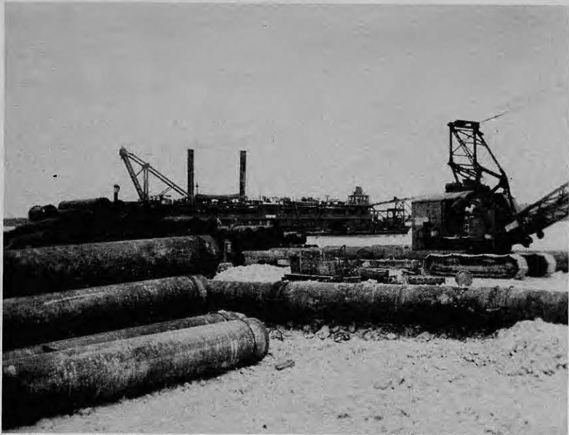
Storing dredge pipe with a crane—the YM-19 in the background
