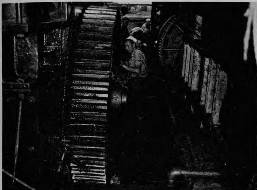
Preparing to remove the main gear
