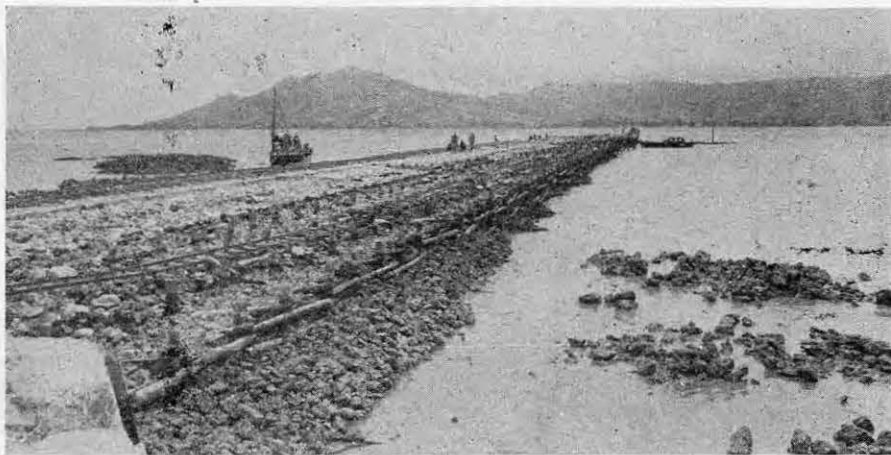
Coral dock at Baten Ko, as left by Japs. Core drill rig is behind pier
