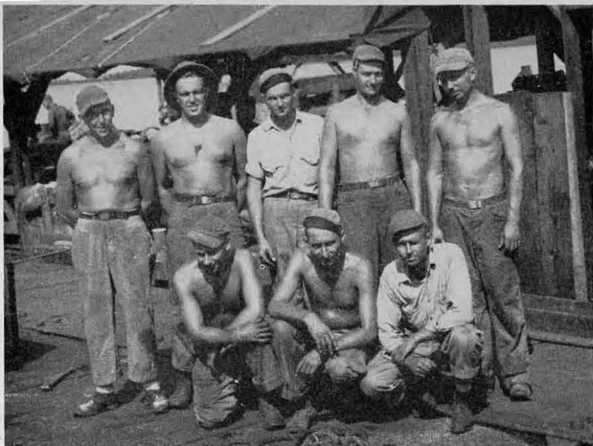
The carpenter shop crew
