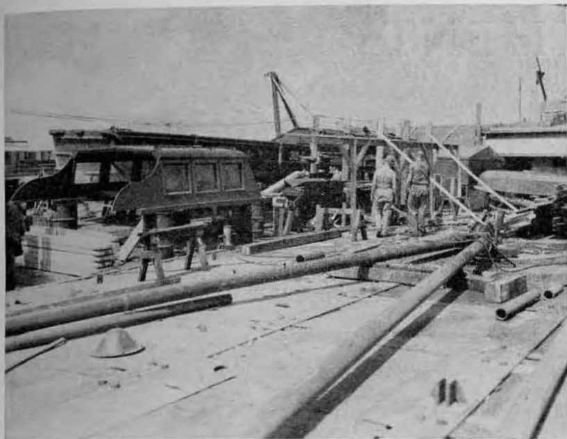
A long shot of the boat repair barge
