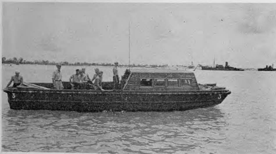
Survey crew sounding from a converted rearming boat
