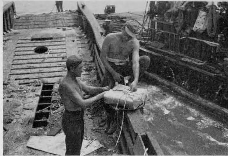
The boys prepare a fifty pound charge to sink an old Jap barge
