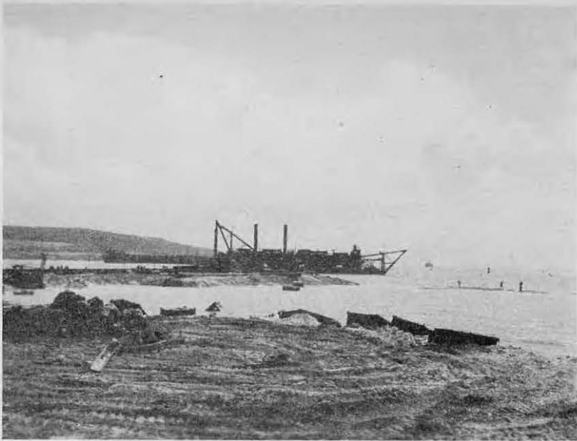
YM-19 Preparing to set up at South Pier
