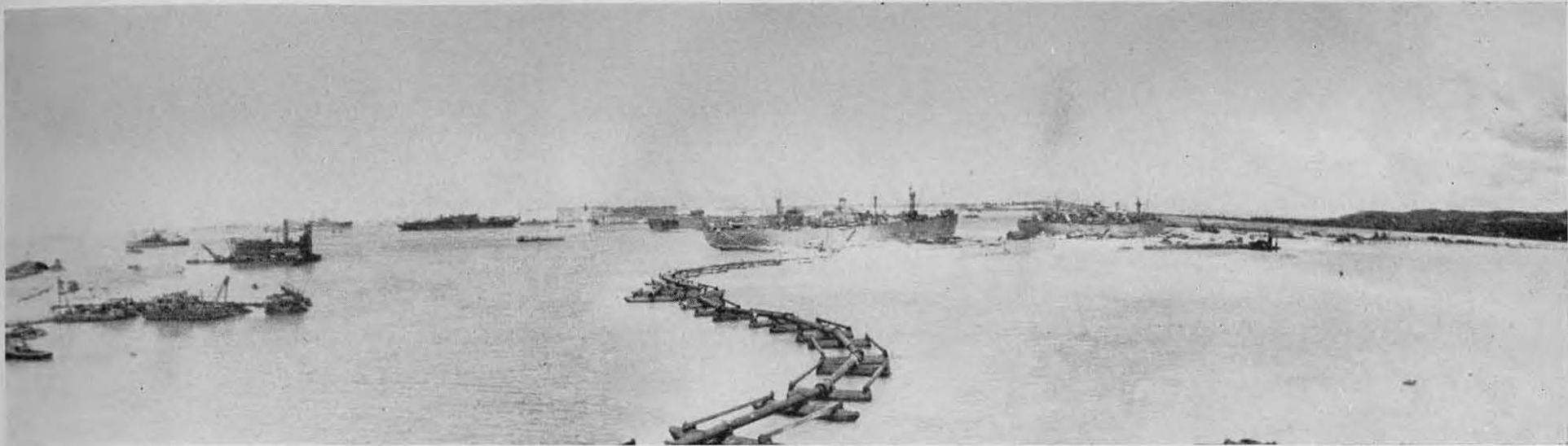
View from the top of a dredge, with the pipeline running to the causeway
