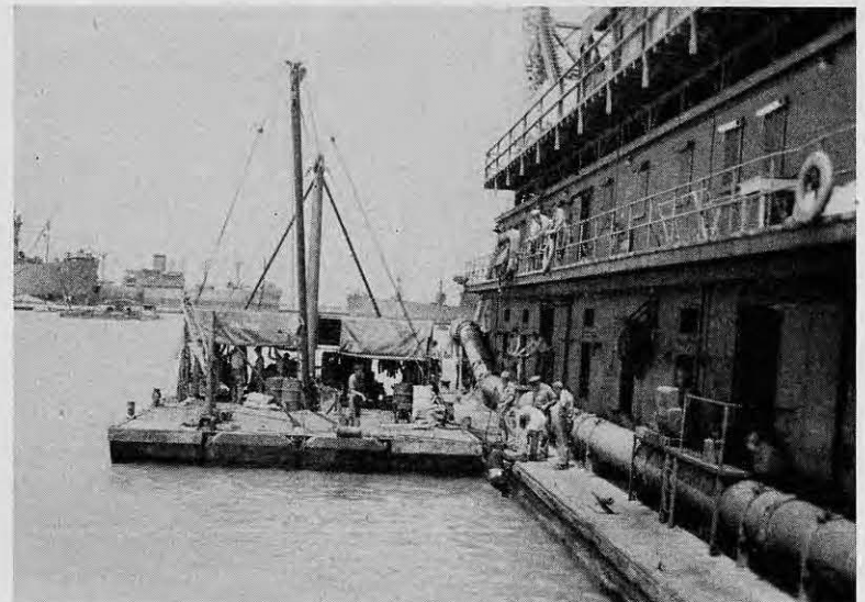
Divers patching hull of YM-18
