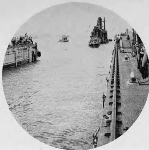
Illustrations of the loading of a dredge in an ARD (auxiliary repair dock). This is YM-19 preparing for a trip from Guam to Okinawa
