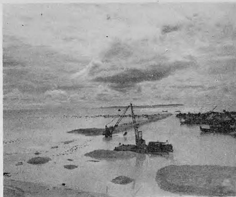
Beginning the Channel
