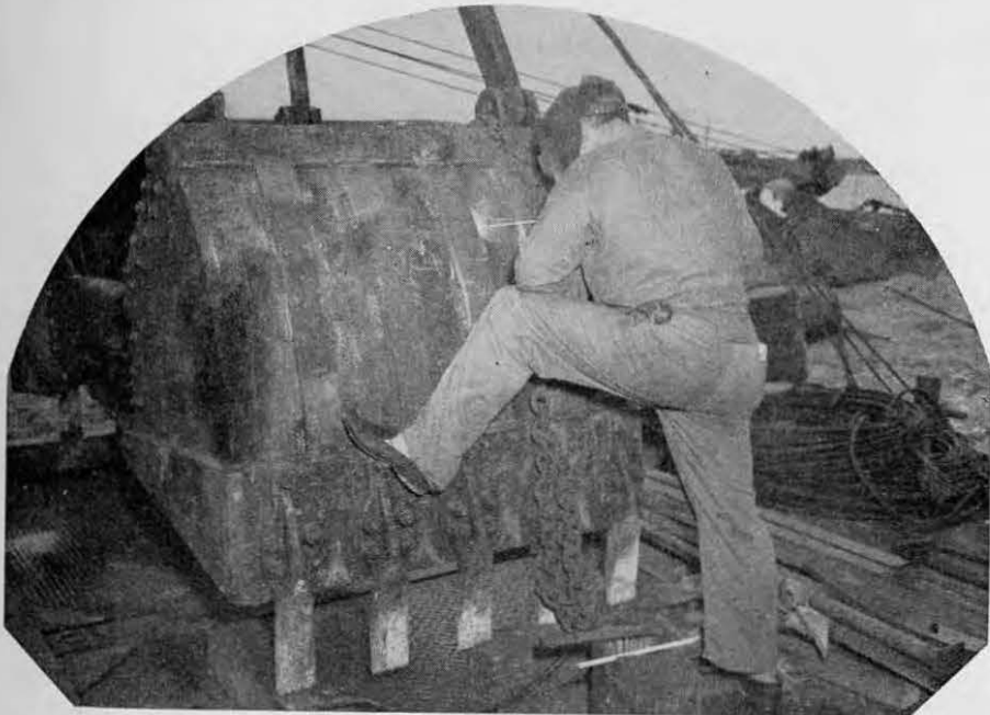
A welder of the mobile unit re-inforces a clam shell bucket
