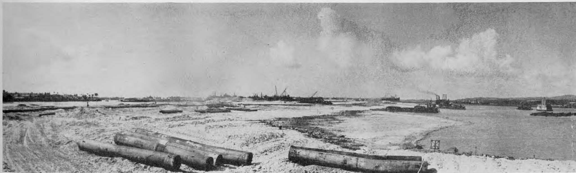
A view of one of the areas our dredges filled
