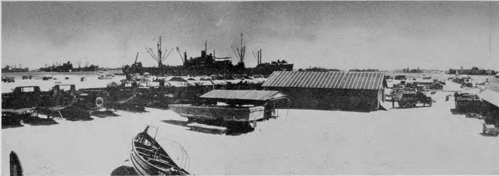
The new boat yard and carpenter shop, with boats on cradles waiting repair or in the process—a busy place!
