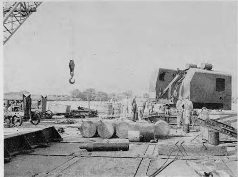
Crane assembly at Aiea
