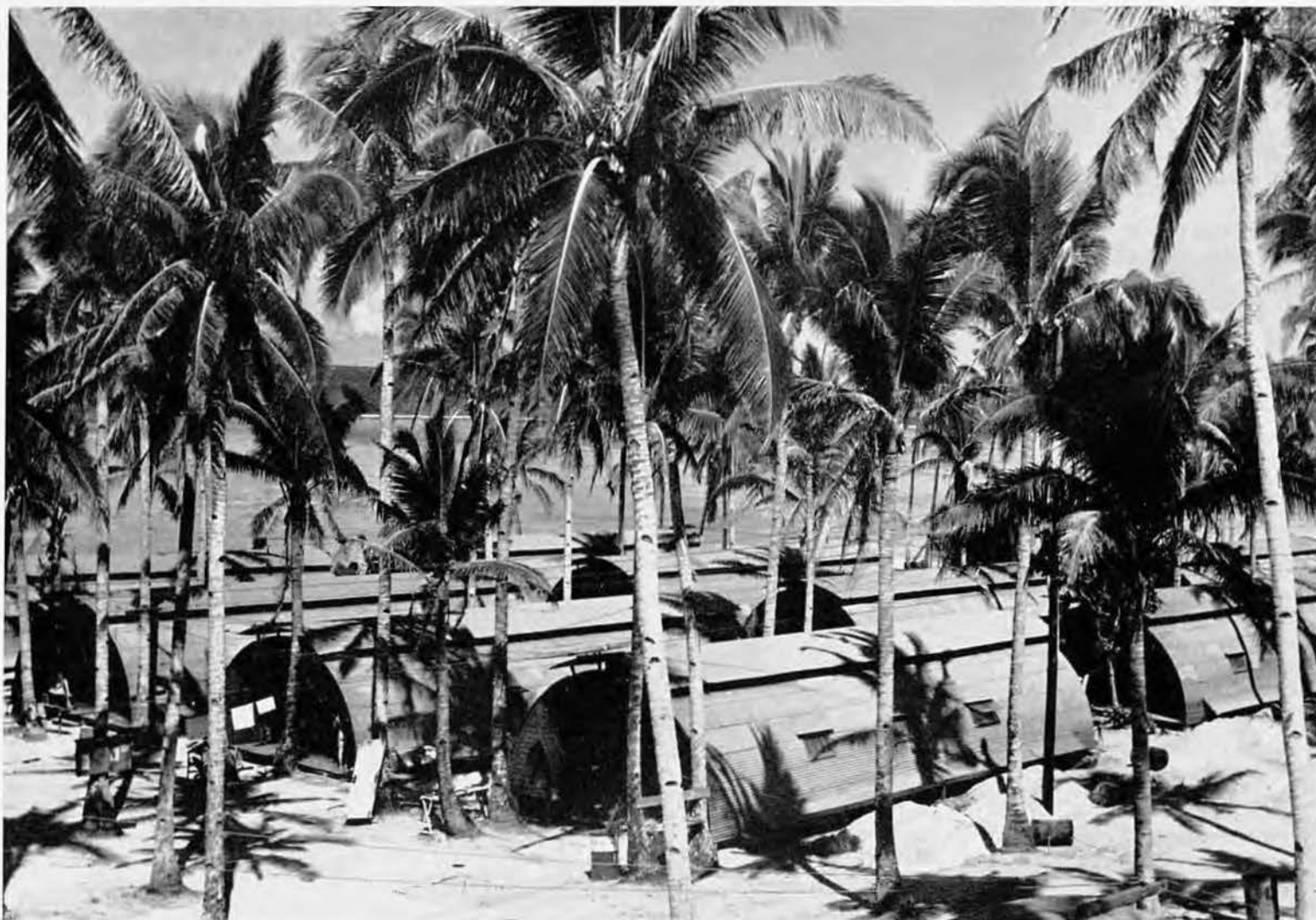
After three weeks of intense work of nine hours a day on the part of the 250 men assigned to camp construction, all except the finishing touches were completed. The following pages are an attempt to give an adequate idea of the finished camp.
