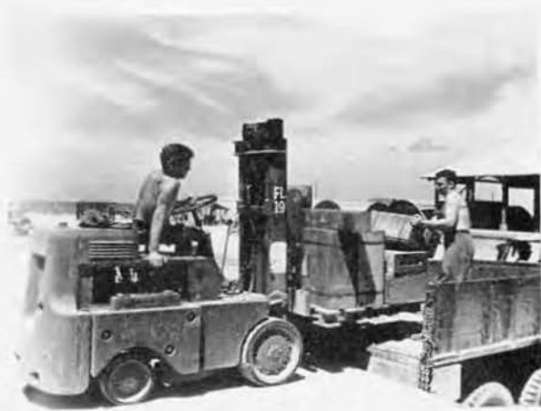
Finger Lift on Loading Platform
