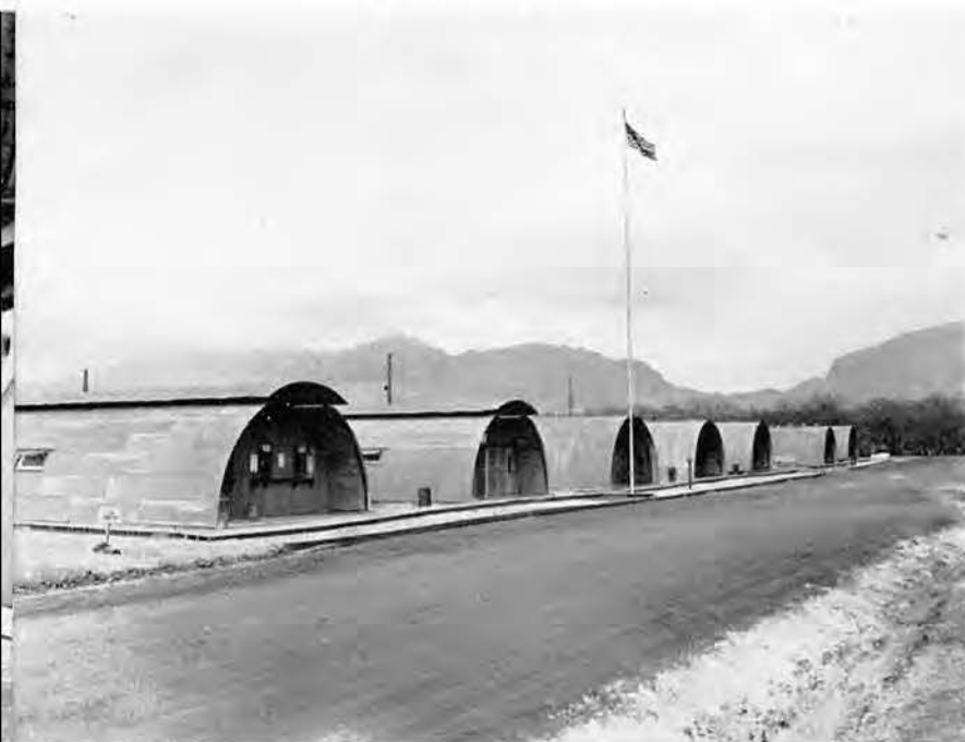
Offices, Camp Dowell.
