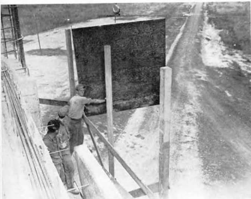
Plywood forms used.
