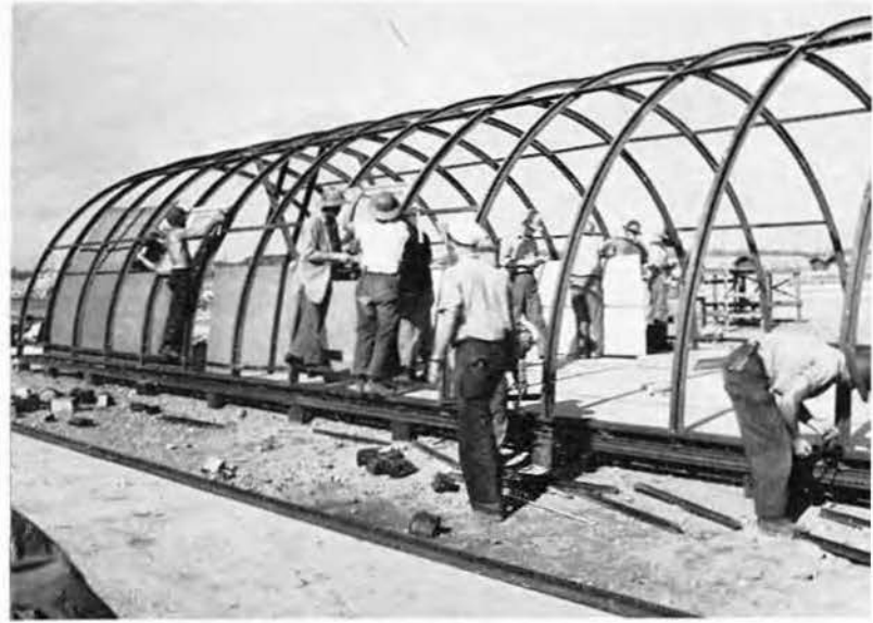
Filling out the ribs.
