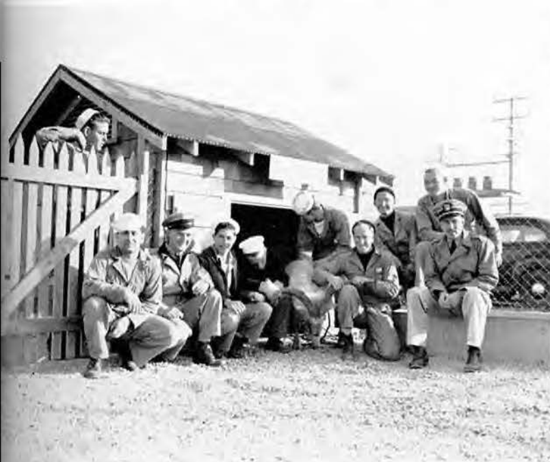
Goat house, our first major construction.
