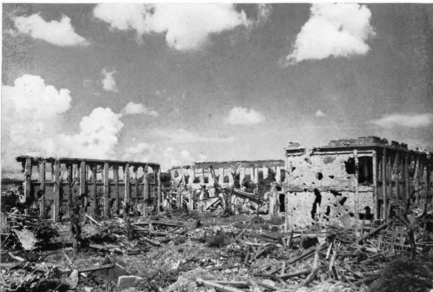
Administrative Building at Shuri
