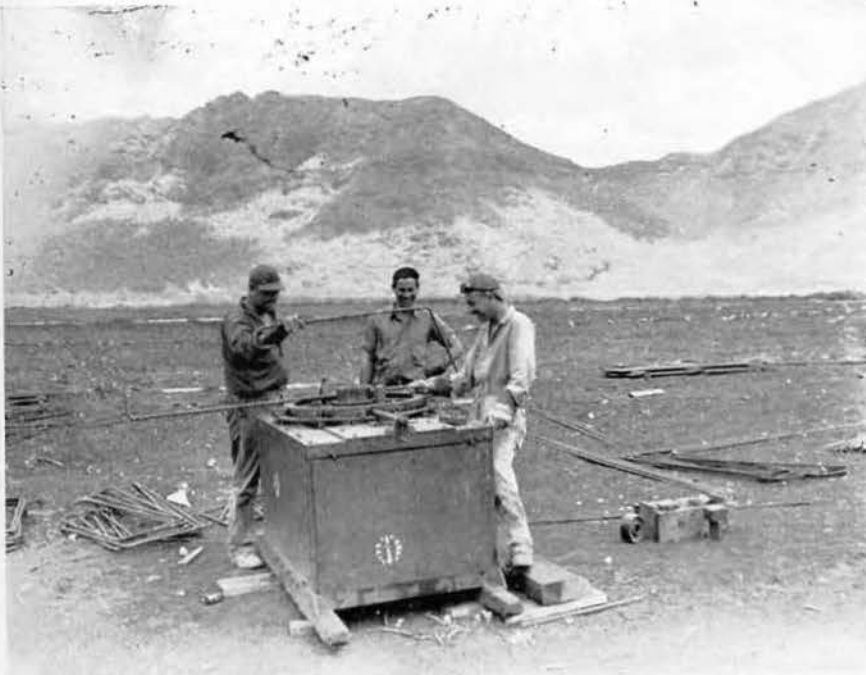
Steel Bent on job site.
