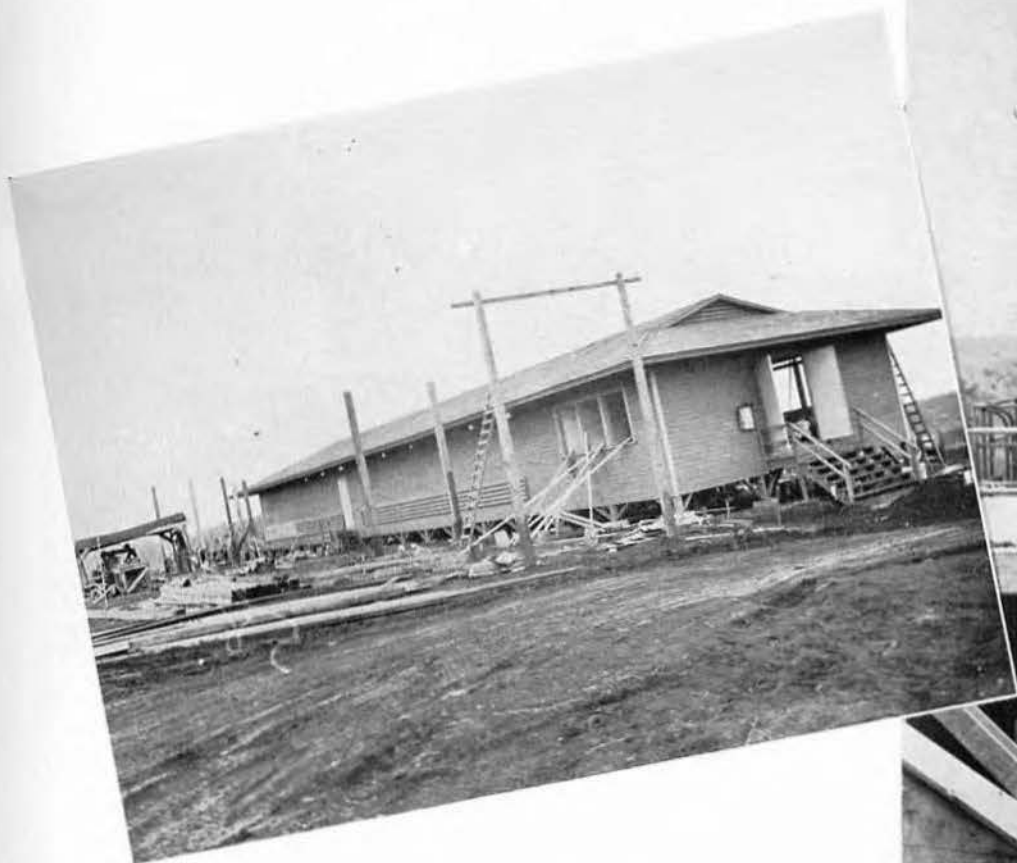
Diversity Receiver building.
