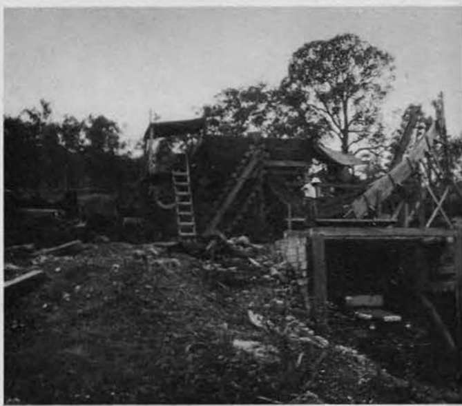
Rock crusher preparing road material
