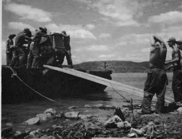
Unloading portable generator
