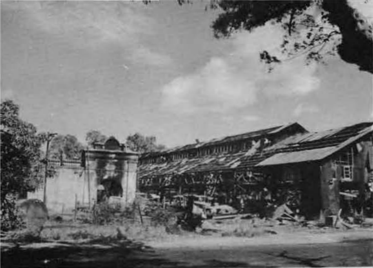
Remains of Power-House
