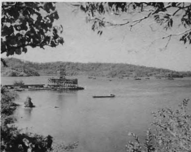
Ship's water supply, the old coaling station
