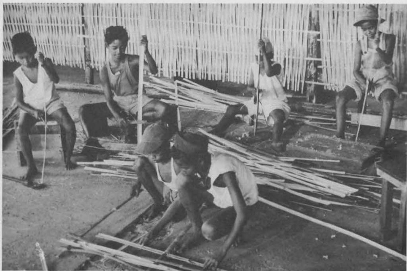
Young bamboo workers repairing Kalalake schoolhouse
