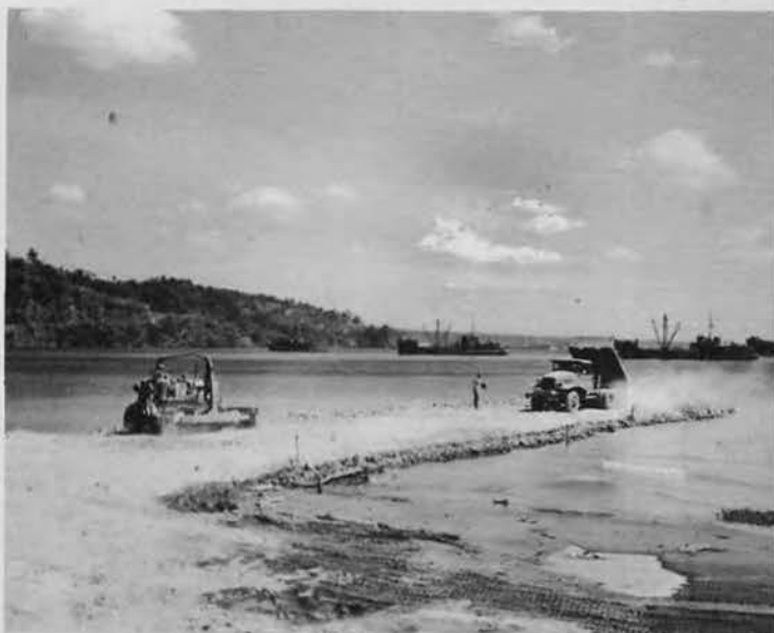
Approach strip . . . Pontoon Dock
