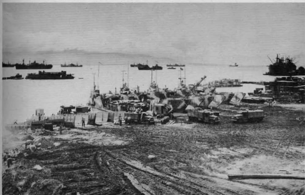
First Project—GAMADODO JETTY
