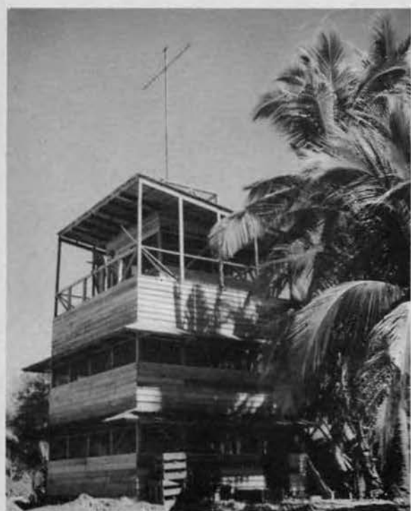
ATC Signal Tower
