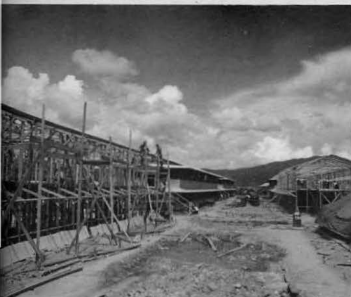
NABU 6 Barracks Under Construction
