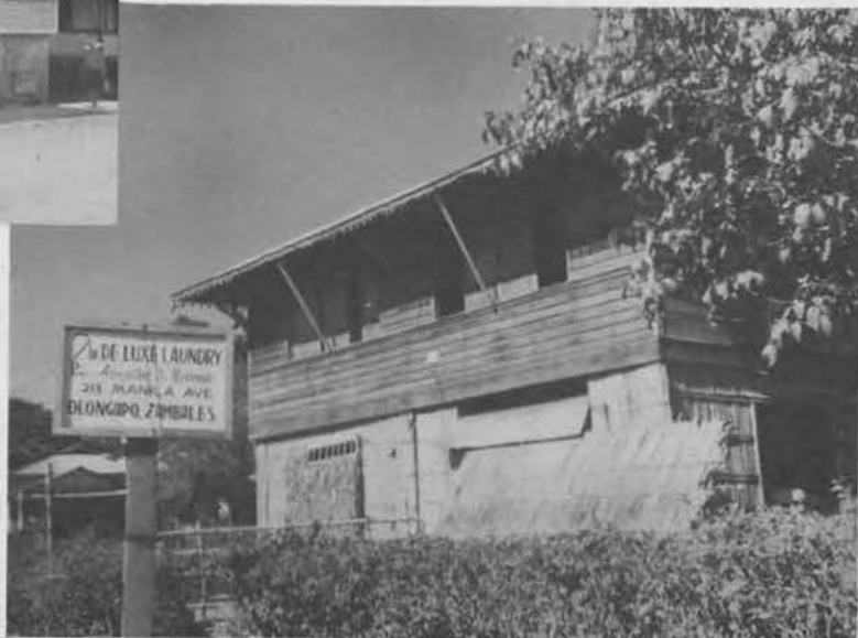
One of the numerous enterprises of this kind
