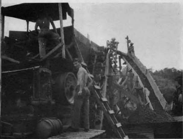
Rock crusher preparing road material
