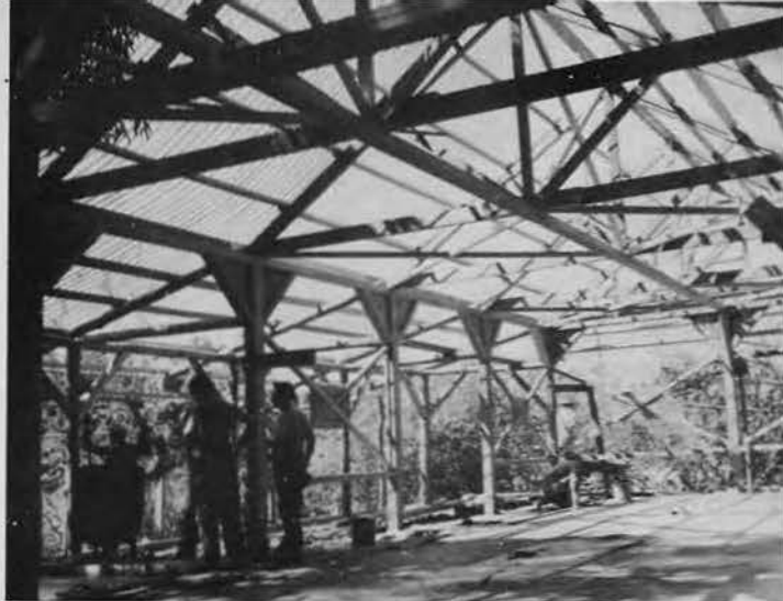
In Process of Construction
