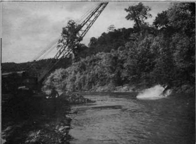
Drag-line working Santa Rita River
