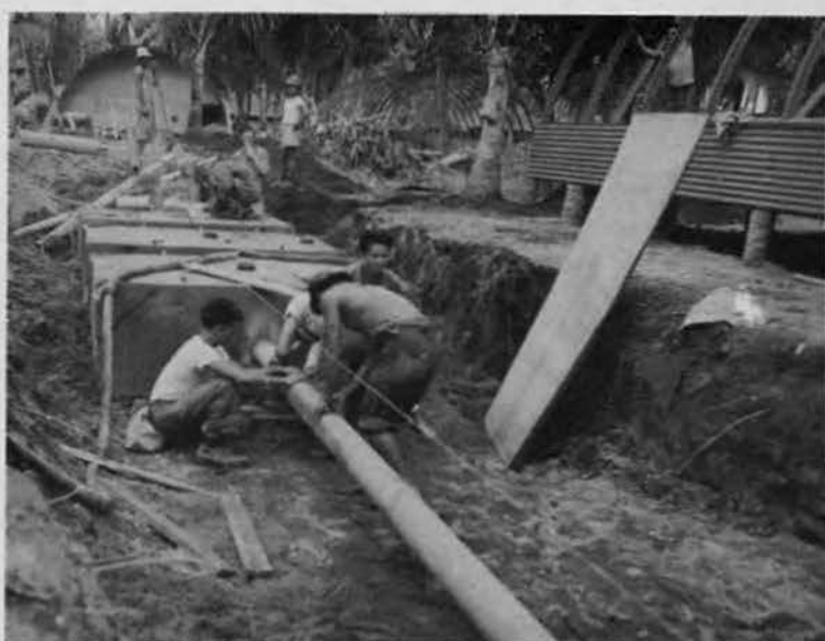
Setting in Septic Tanks
