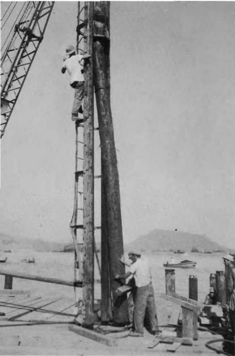
Placing piling in the leads of the land pile driver.
