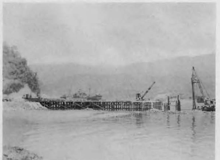
Left: Hill drops sharply to water at Destroyer Cove in May '44. Right: Hill is hacked away for road, dirt ramp and partially finished Destroyer Dock extend into cove 9 weeks later.
