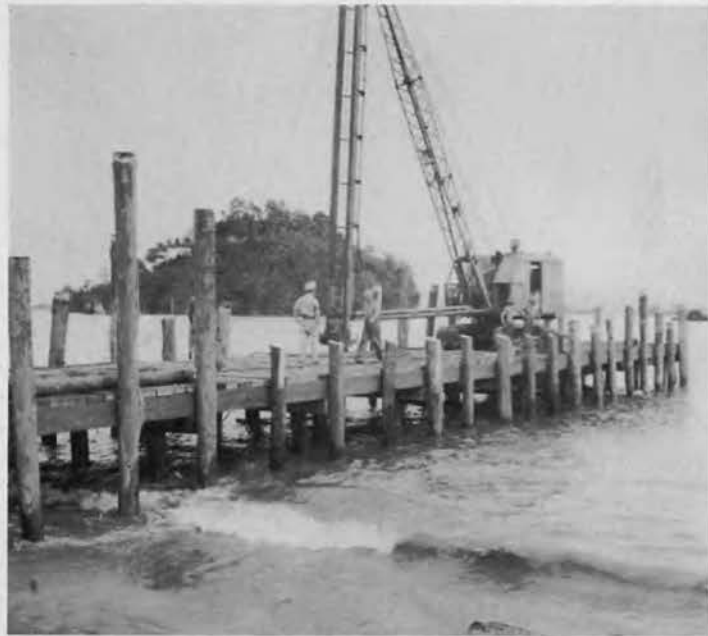
Driving fender piling on the substantially completed Small Boat Dock.
