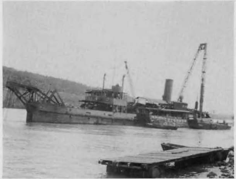
Dredge D. York Syme opens channel for Small Boat Dock.
