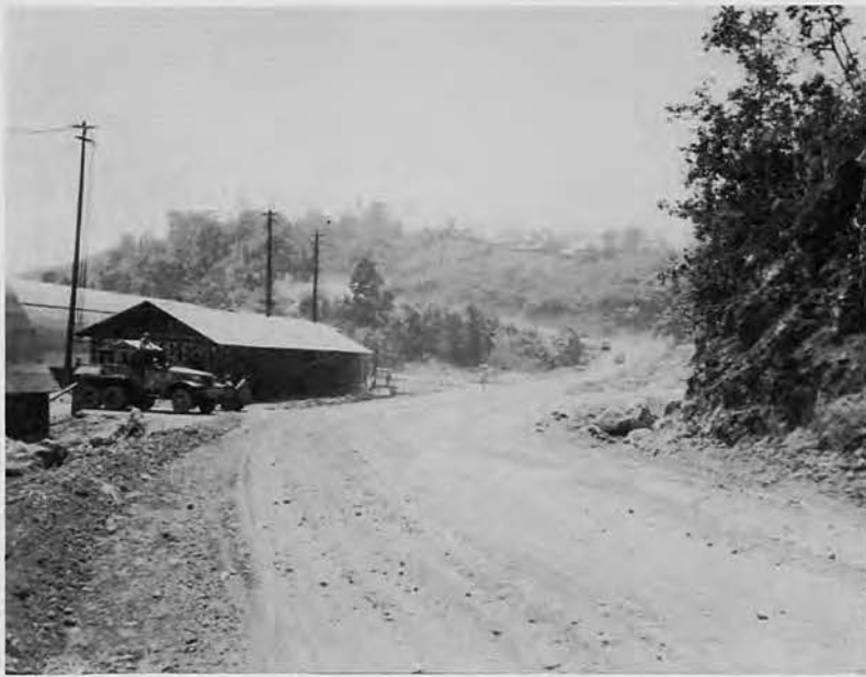
Generator Bank (in building behind truck) installed by 113th Electricians, supplied light and power for docks, shops, forges of Destroyer Repair Base.
