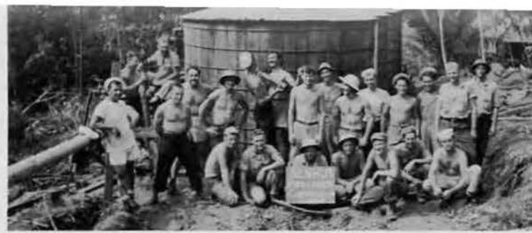
Pipe Line Crew pauses for poses at completion of water supply line to 113th Camp.
