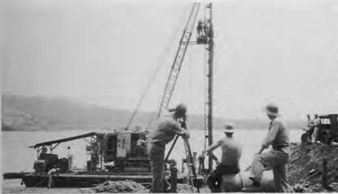
Survey Crew locating the first piling for Hollandia's Navy Dock No. 2.
