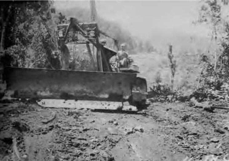
Cable-rigged 'dozer begins one of the many tributary roads in Hollandia.
