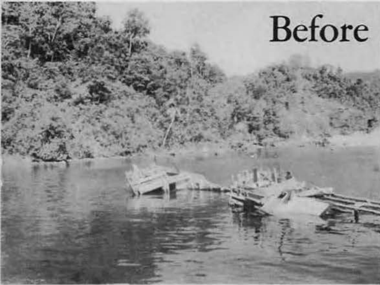
Left: Jap barges impaled on coral reefs. Right: Few weeks later, dirt fill covers barges and reefs. Dock No. 1 is complete enough to unload and water Liberty Ship.
