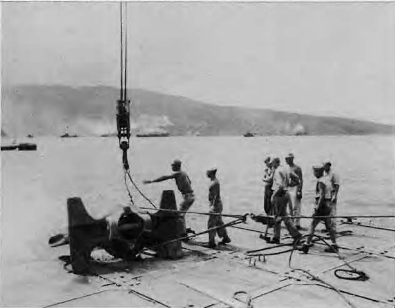
Rigging Crew setting the anchor for cruiser mooring buoy.
