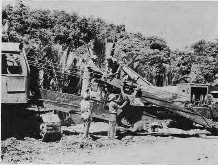
Above: Heavy Equipment Riggers at Hollandia rigging a Northwest shovel.
