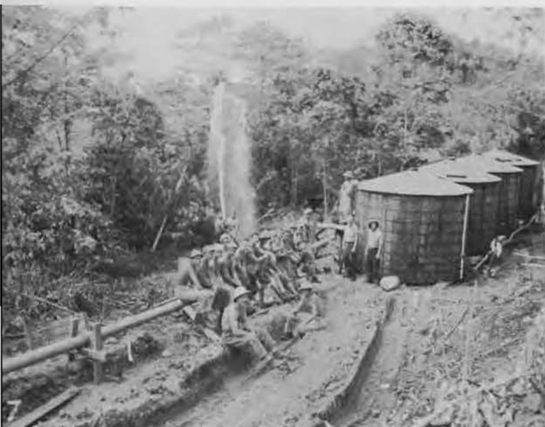
Above and below: Pipe line crew tests final connection of 5,000 foot line to 113th Camp tanks of 5,000 gal. capacity each. Dirty Seabee revels in first shower since landing.
