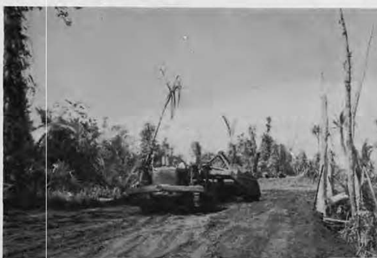
To the north of Pancake Hill part of the vast Sago Swamp was filled in for a Staging Area and Supply Dump. Carryalls in a constant procession brought earth and rock from ramps cut into Pancake Hill.
