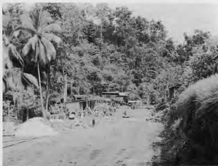
Reefer Banks (left center and center background) of Carrier knock-down units, first installations in 113th Mess Hall Area, were immediately crammed with fresh meats, fruits, vegetables.
