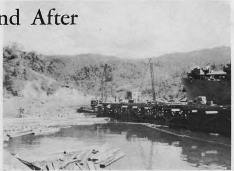
Left: Jap barges impaled on coral reefs. Right: Few weeks later, dirt fill covers barges and reefs. Dock No. 1 is complete enough to unload and water Liberty Ship.
