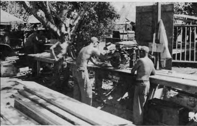
Production experts prefabricate tent frames and floors with saw powered by portable generator in center background.
