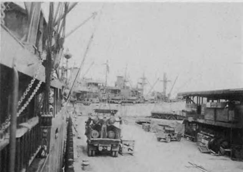
Unloading operations on Navy Dock No. 1 are in full swing. The Rigging Loft addition at the right is shown completed. In the background a cargo ship is tied up at Dock No. 2.
