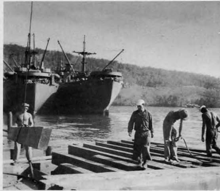
Installing stringers for the Hollandia Small Boat Dock.
