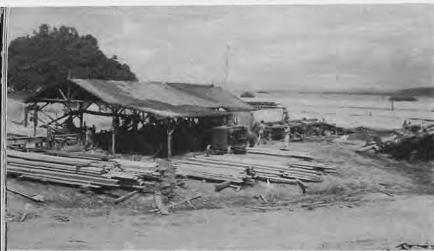
113th Sawmill at Pie Beach, Hollandia, was assembled from salvaged Japanese equipment.
