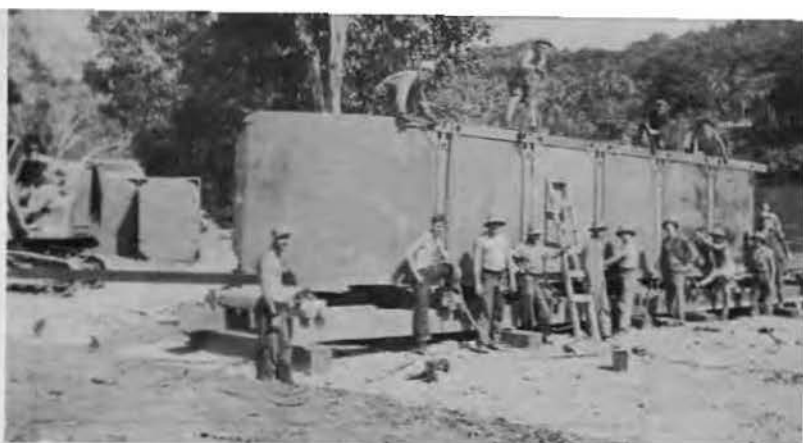
Assembling pontoon barges.
