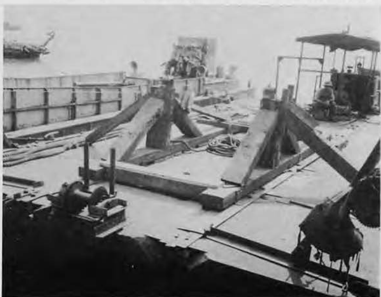
Close-up of the pontoon barge rigged for underwater cable laying operations.
