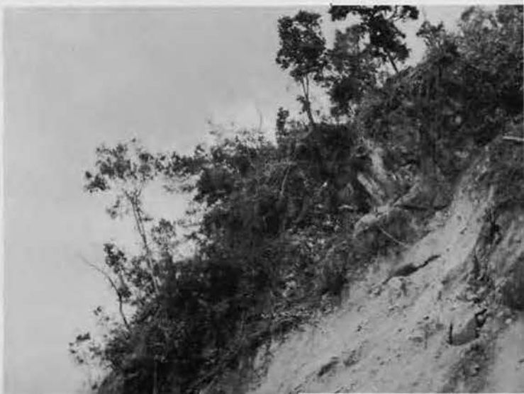
Typical of dozens of spot blasting jobs in Hollandia road construction is this overhanging rock near Dock No. 1.
