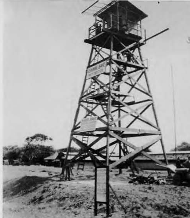
Port Director's Signal Tower, one of first structures built by Detachment "C", commands Mangarin Bay, outlet to South China Sea.
