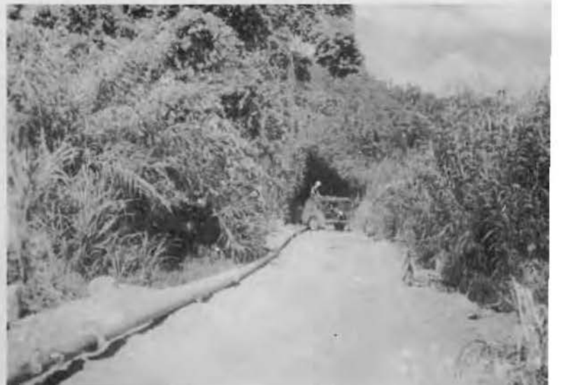
Temporary water line and pump at Hollandia Spring.
