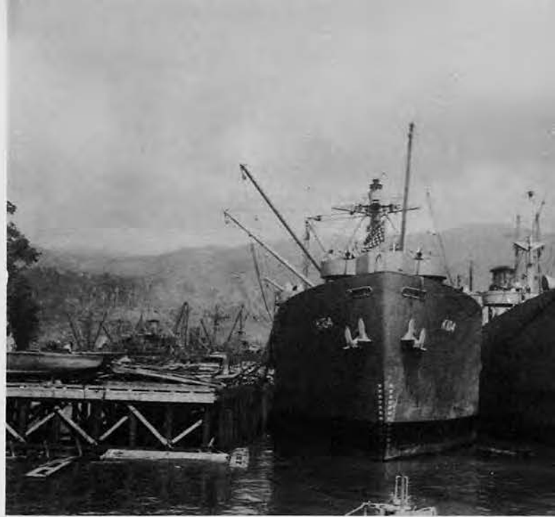
Dock No. 2 before completion.
