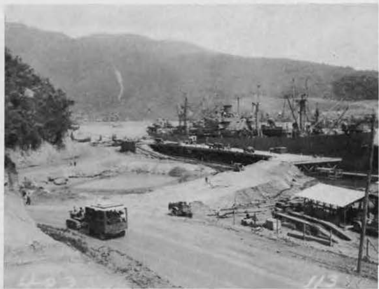
Left: Proposed location of Navy Dock No. 2. Right: Hollandia Road snakes along dynamite-leveled shoreline; approaches are built to completed Dock; center area will be filled, Sorting Docks built to expedite distribution of cargo.
