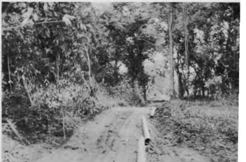
Water pipe laid along proposed line after 'dozers cut road through
