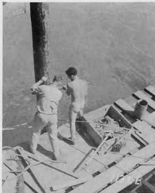
Adjusting piling preparatory to driving.
