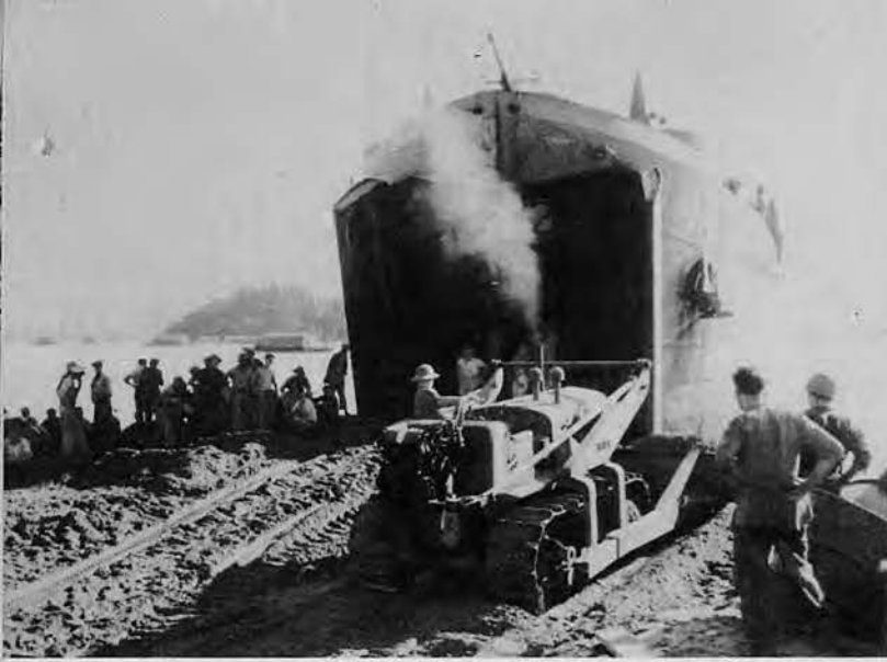
Bulldozer constructs ramp for loading LST, the ill-fated 472 (see frontispiece).
