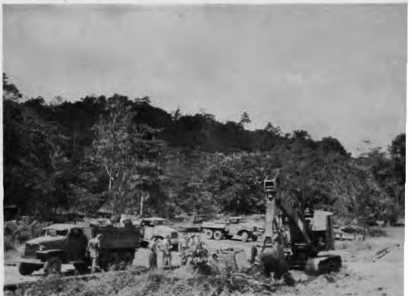
Backhoe digging trench for Base water supply pipe line.
