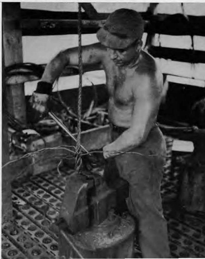
Making a splice in a cable at the Rigging Loft.
