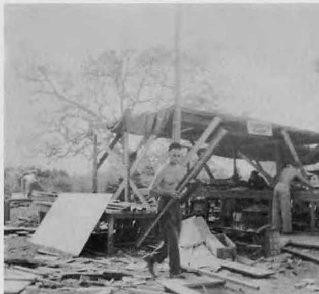
Detachment "C" Carpenter Shop, center of building construction activity on Mindoro.
