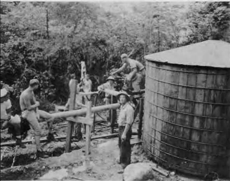
Above and below: Pipe line crew tests final connection of 5,000 foot line to 113th Camp tanks of 5,000 gal. capacity each. Dirty Seabee revels in first shower since landing.
