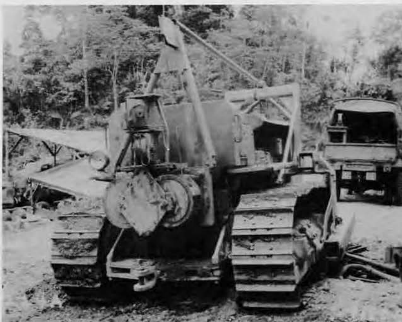
Standing on corrugated metal roofing which offers only slight protection against the mud, Heavy Equipment Mechanics A. A. Goste, and F. F. Schade push repairs on a bulldozer outside the Mindoro shop. Chief H. H. Nickels watches progress of the job.
