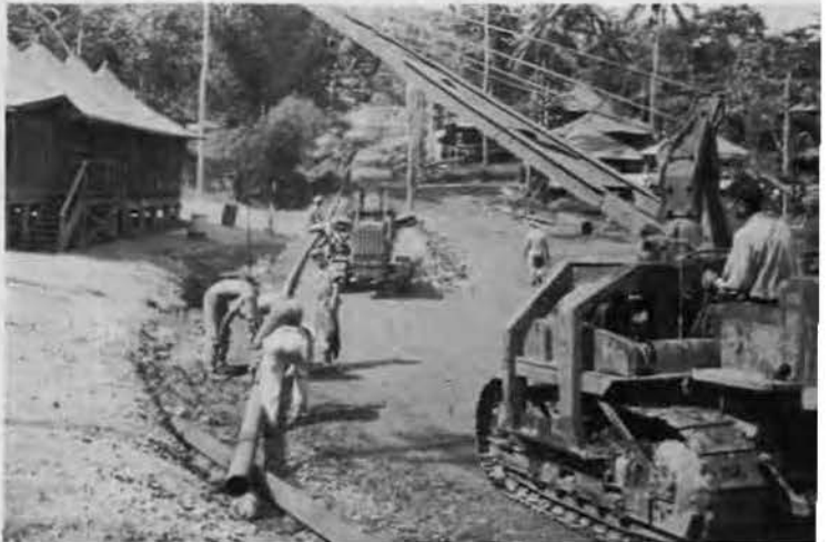
Digging ditch and laying 6" pipe through 113th Camp Area.
