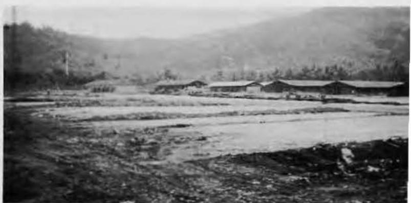
Warehouse and reefer building construction at Naval Supply Depot.
