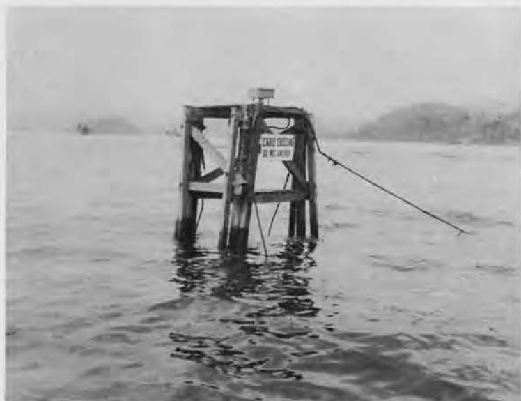
Pile dolphin for terminal box on underwater telephone cable installation.
