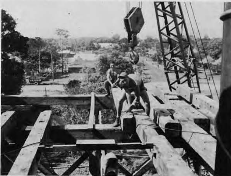
Riggers place heavy timbers in water tank tower construction at Mindoro.
