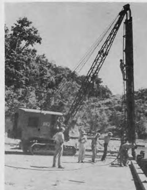
Driving the fender piling for Dock No. 1.
