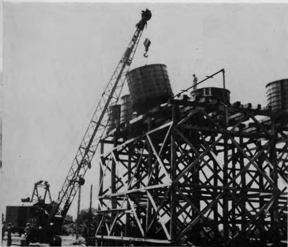
Frame of 5,000 gal. tank is set in place on water tower at Mindoro.
