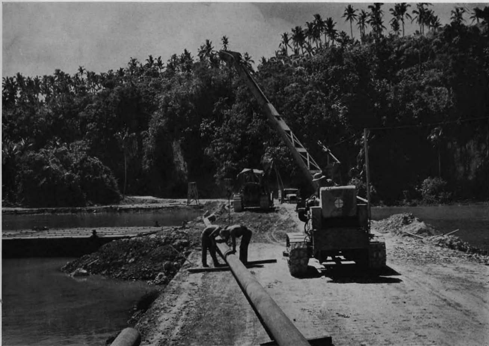
Pipeline Project Over Causeway
