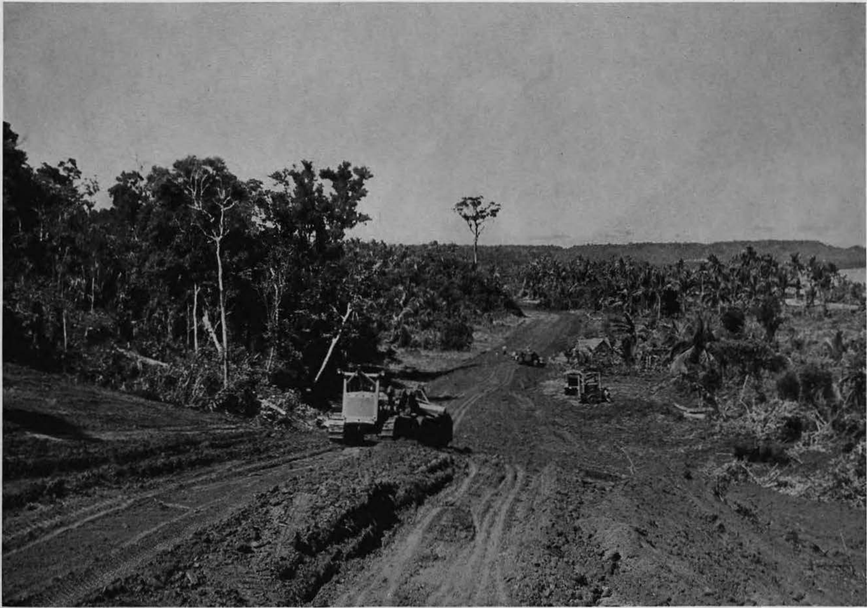
The Road Progresses
