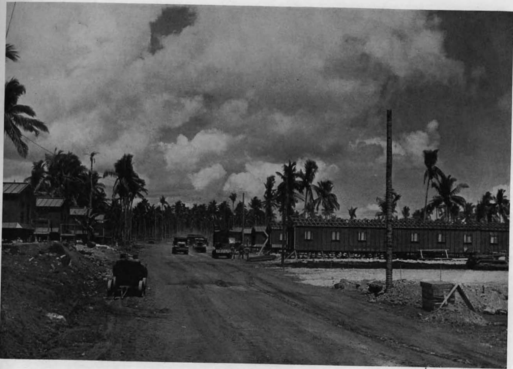
Hospital Project FLEET HOSP. + AT # 114
