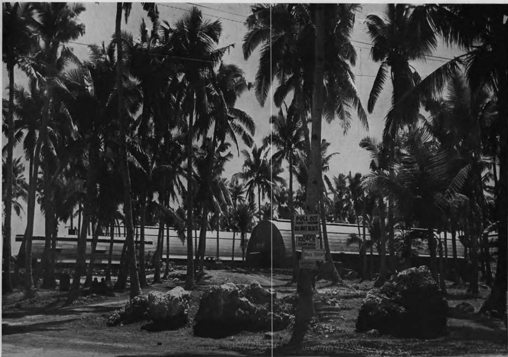
Administration Area, "After"
