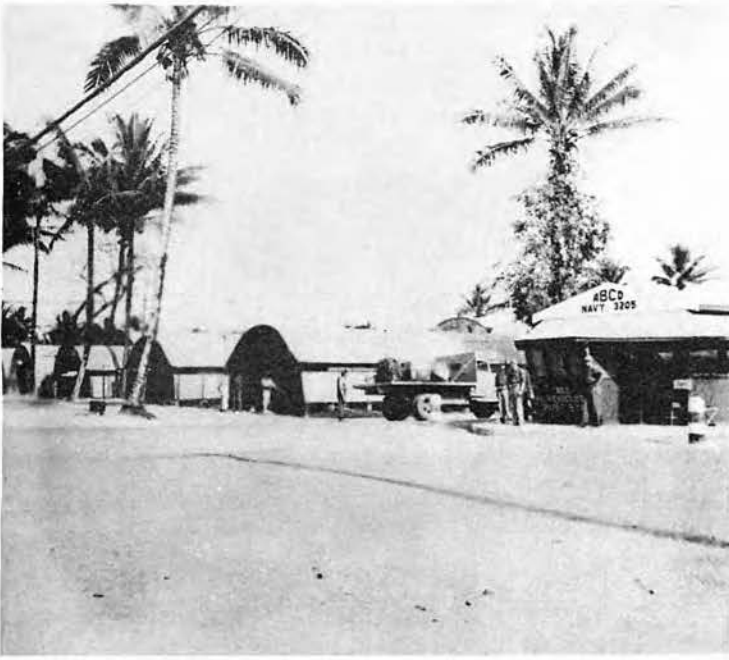
A truck is checked in at Gate No. 1 . . .
