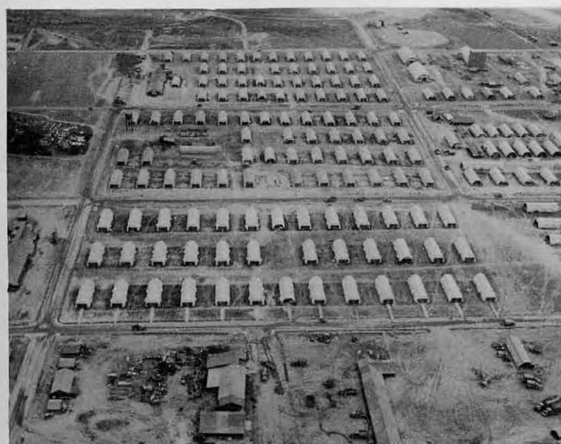
AERIAL PHOTOGRAPH taken 29 June 1945 from a northern approach showing the huts utilized for housing at the USN ACORN 34 base command camp area, Clark Field. Enlisted 1200 man galley and mess hall No. 2 with chief's mess is at upper left corner of camp area. The storage tank beyond galley is a 1000 bbl. steel tank used for water storage supplying the 15,000 gallon wood stave tank located to the right of the Filipino village. In the foreground are various shops including electrical, carpenter, refrigeration and paint shops at left foreground; garage, plumbing, welding shops in center foreground; civilian labor distribution shed at right center.
