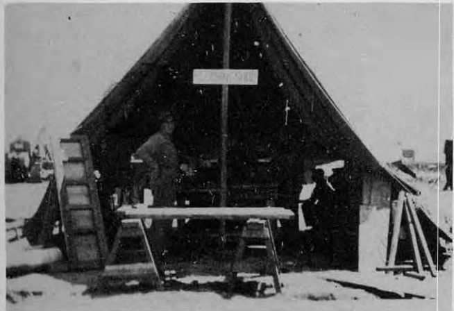
PLUMBING SHOP. Chief Grasso (shown here) and his plumbing crew installed all camp water lines and showers.
