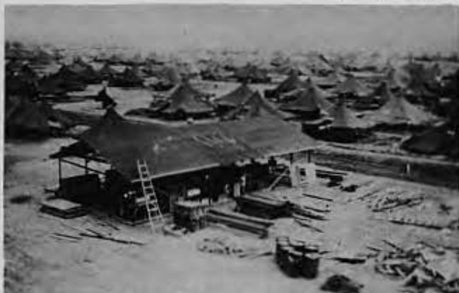
AIR VIEW OF NAVAL CAMP AT MANGALDAN, LUZON, P. I. CBMU 606 carpentry shop is shown in center foreground, temporary mess tents are at left, and temporary tent quarters for personnel are in the background.
