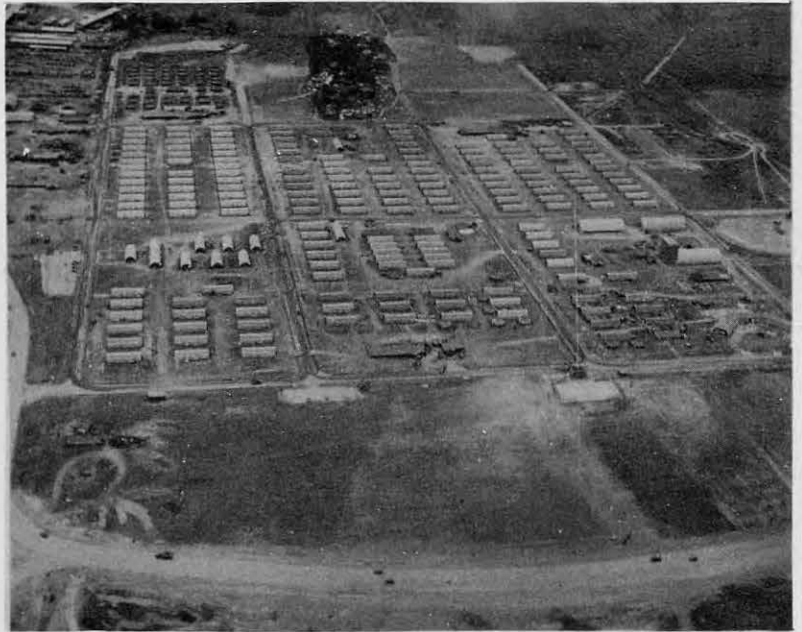
NAVAL CAMP, CLARK FIELD, 29 JUNE 1945. Stran Steel Huts have replaced temporary tent quarters and administration buildings, with the exception of the Sea Bee quarters. Men of CBMU 606 evidenced a marked preference for tents rather than prefabricated huts for housing.
