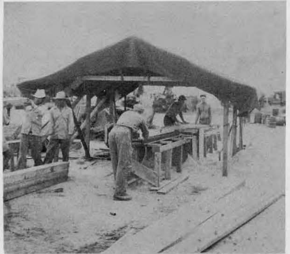
CBMU 606 POWER SAW. Being operated by Hart, Morgan, Gunderson, and Haman.
