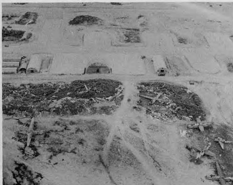
AERIAL PHOTOGRAPH of northern end of taxiway No. 3 at Clark Field showing construction by CBMU 606. Huts at extreme left include two ordnance buildings, one office, and one quick engine change shop with a smaller hut serving as a generator building. The canvas covered building at center is a 78 feet by 30 feet nose hangar, and the hut at the right of the picture houses a radio and radar repair shop. (Note destroyed Jap planes in foreground.)
