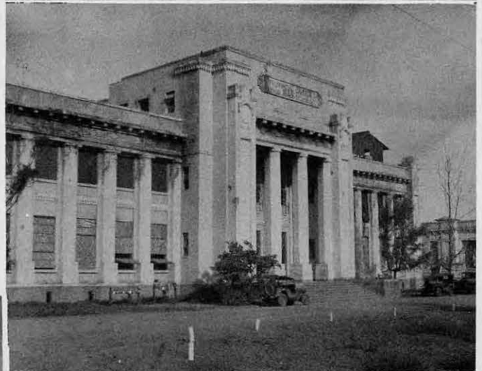
MALOLOS — This Bulacan provincial capitol building at Malolos was a familiar landmark to all Sea Bees heading to Manila for liberty. Built in 1935 the building housed Japanese militia during the occupation and was thus subjected to bombing by the American Air Force on January 12 following the Luzon invasion. Damage was not extensive and the capitol is now used jointly by the Provincial Board and the Military Police Command.
