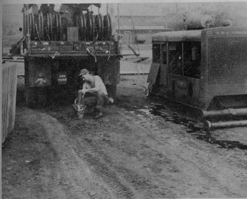
SERVICING THE GENERATOR
