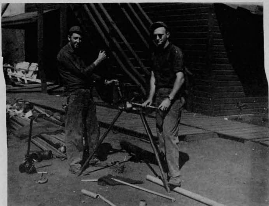
THREADING PIPE
