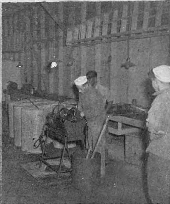
Plumbers at work
