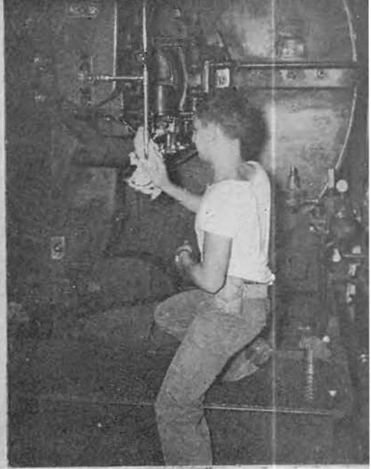
Wiper in the Evaporator Plant
