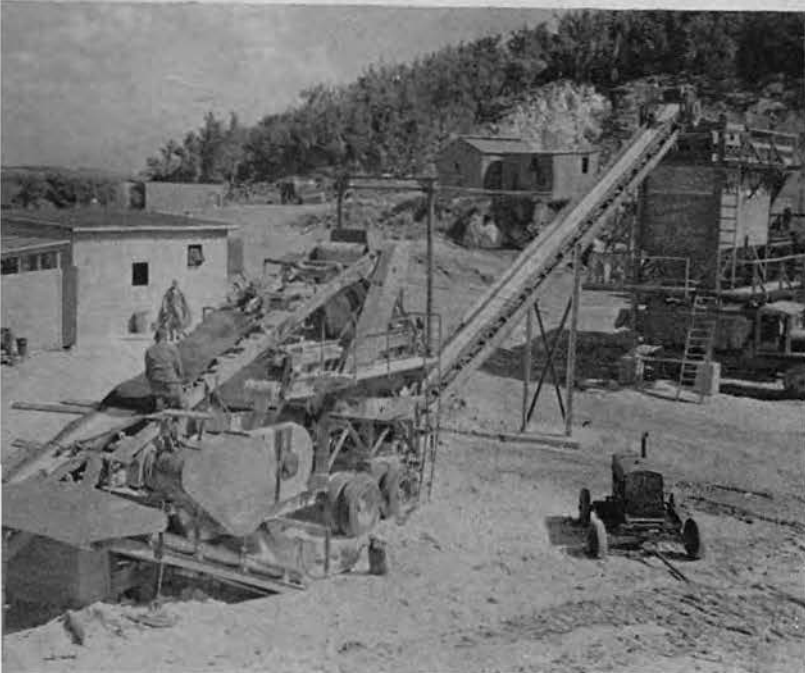
Rock Crusher and Quarry, Harrington Sound, Bermuda Road Project
