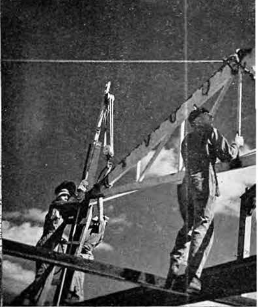
Setting roof truss
