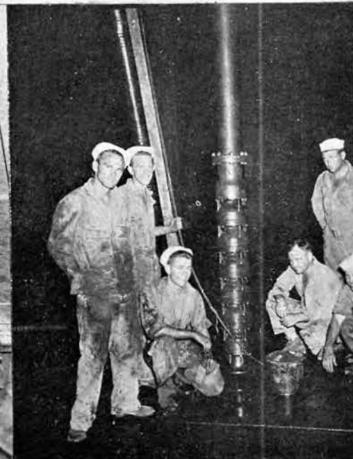
Fuel Oil Maintenance
