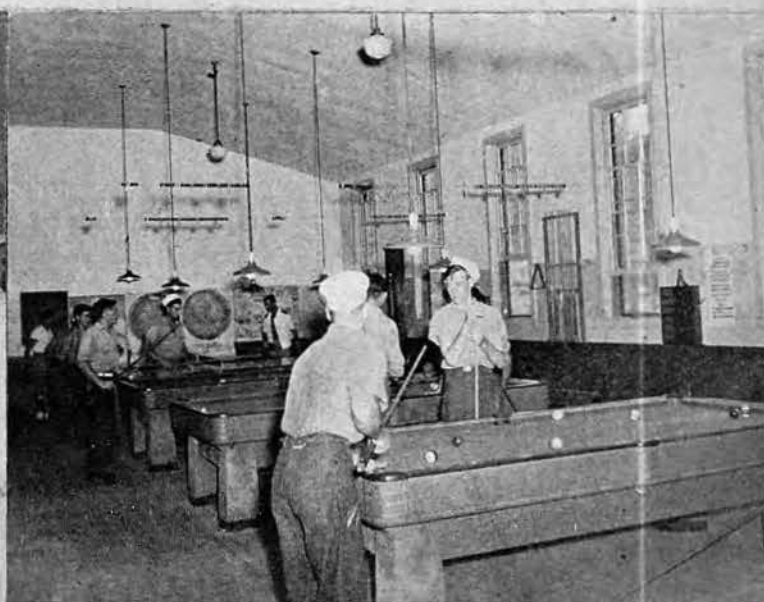
Pool hall in the Recreation Building
