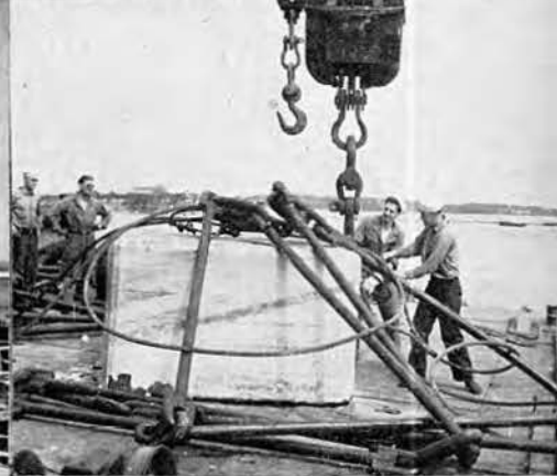
Setting Buoy Block
