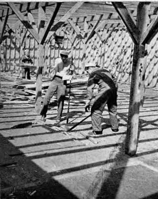
Tearing dunnage from Warehouse
