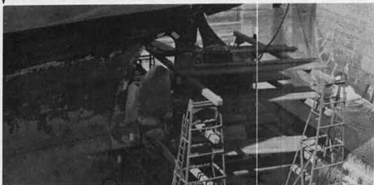
SCAFFOLDING UP ...Repairs begin
