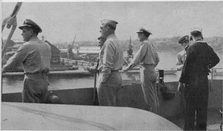
CAPTAIN ON SIGNAL BRIDGE ... .... Keen eye on entering drydock
