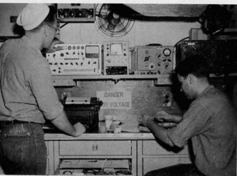
CHECKING INSTRUMENTS IN "ET SHACK"
