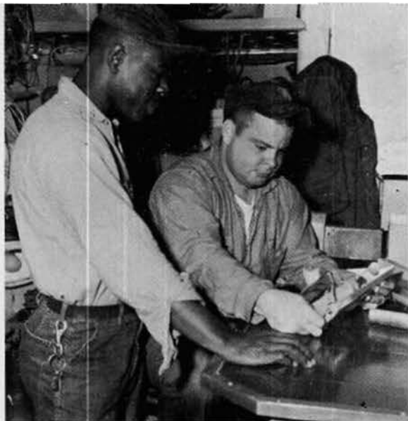
ELECTRICIANS AT WORK
