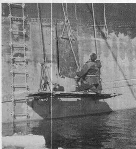
STEEL BANDAGE ... Repairman at work on ice-smashed hull
