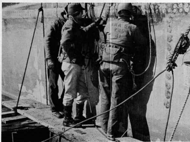
FINAL CHECK BEFORE CAPE HALLETT DEPARTURE
