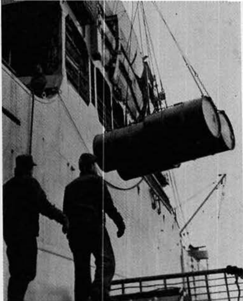
LOADING OIL DRUMS
