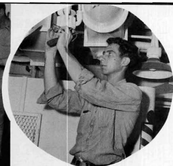
Light Repair Near Barber Shop
