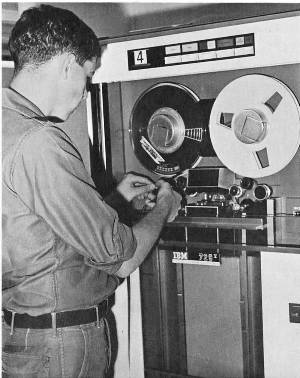
1 | 2 DP2 R. J. Studer threads an IBM 729 Magnetic Tape Unit.
