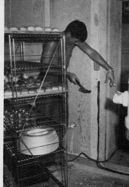
Bake shop, SEABEE installed.
