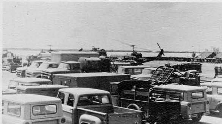
302 constructed helo pads in background.
