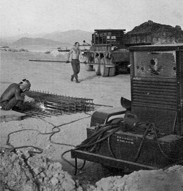
Early morning dawn finds steelworkers already hard at work.
