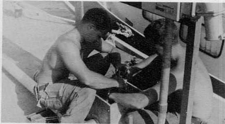
CE's splice 440V pier power, CRB.
